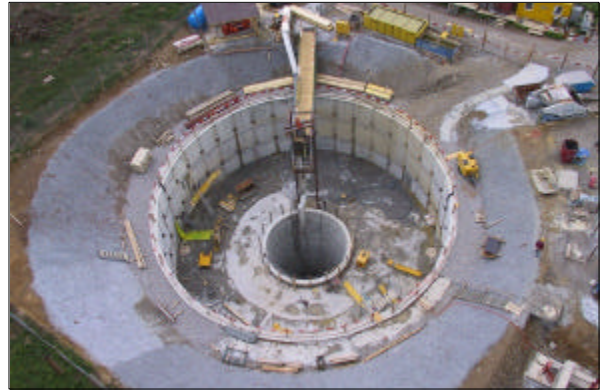
Ventilation shaft and construction pit for chimney foundation
