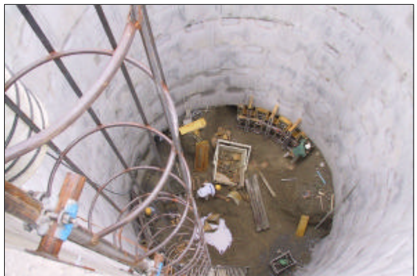
Shaft construction in soil section (underpinning)
