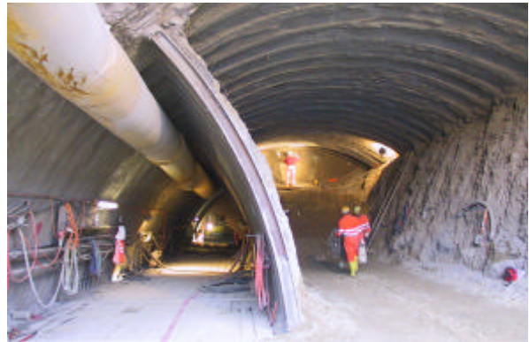
Core boring with steel installation
