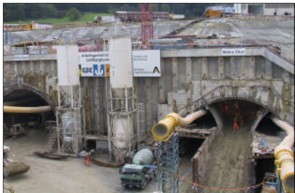
Reppisch valley excavation (Portal Diebis stand June 01)
