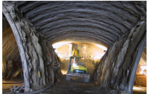
Core boring with steel installation
