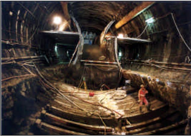
Core method of construction in all soil sections (example Diebis)
