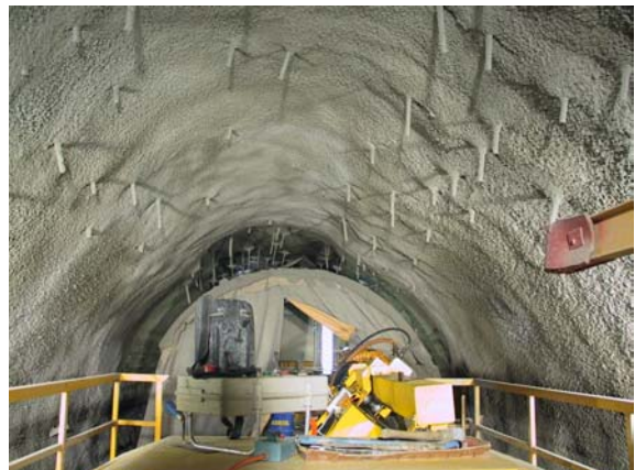
Pilot TBM with rock support
