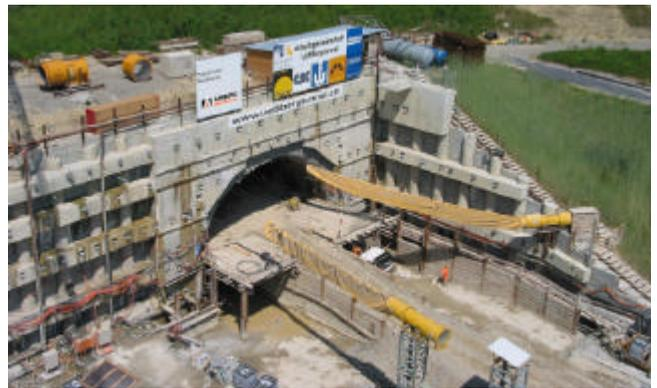
Fig. J: Portal view of the Gänziloo excavation site / driving the Juchegg soft ground section
